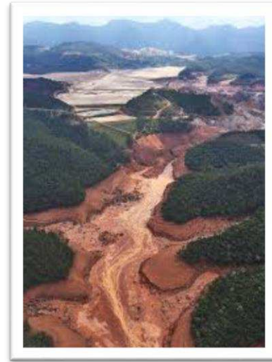
Fundão dam collapse
